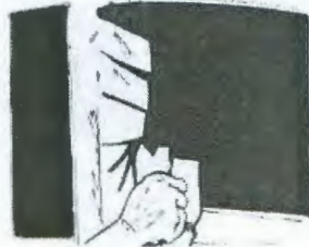
7. Cuts are made at curves of window opening and between for a good fit. Material is then pulled around window lip and glued down.
